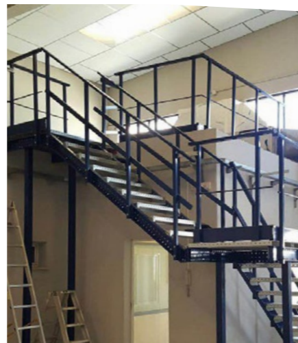
STAIRCASE WITH LANDING
